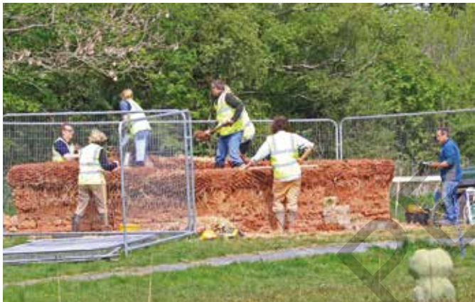
Volunteers learning clay dabbin construction skills
