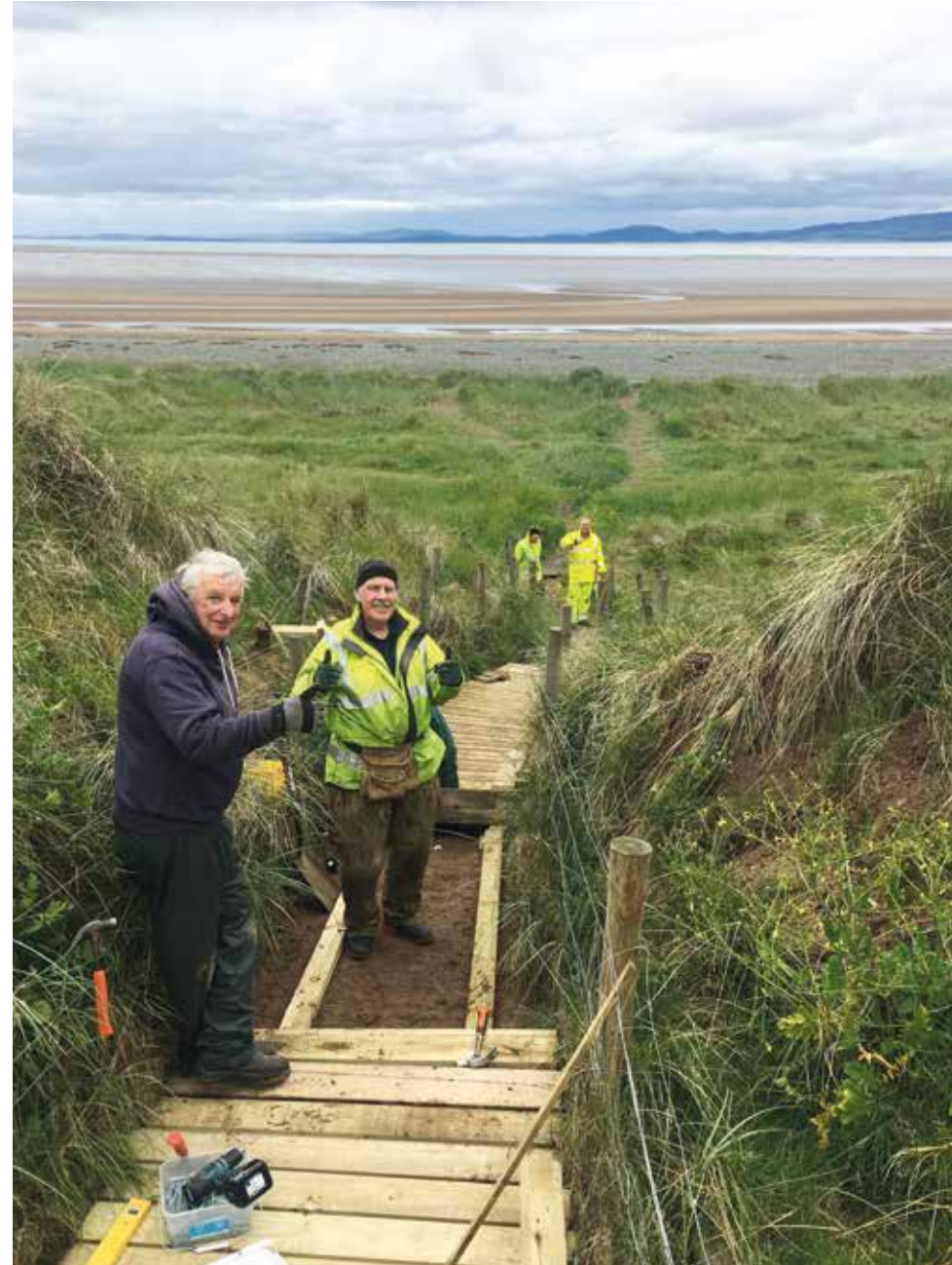
Hard working volunteers constructing a new visitor boardwalk at Wolsty Banks
