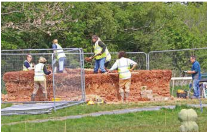
Volunteers learning clay dabbin construction skills
